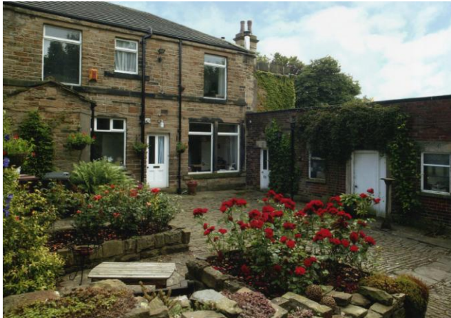
Left: 1. Sowood House North aspect 2003 The side facing north. The block on the right is the old dispensary block, the upper floor being removed in 1948. The brick facing was probably added later, but before 1937. Note the windows are “squarer” than those at the front and were originally with sashes. The stone setts in the courtyard and drive were the original ones and were never re-laid.
