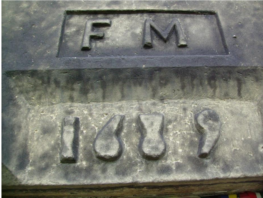
Datestone above the door at Sowood Farm (October 2012)
