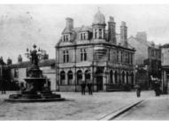
With its distinctive dome, the old Midland, then HSBC Bank was one of the most recognisable and iconic buildings in Ossett and was built in 1891 for the London City & Midland Bank. In September 1958 the dome was removed due to the interior structure breaking up and stone from the inner core of the dome falling into the living accommodation below. The building was sold in 2020 and the top floors have been converted into three
