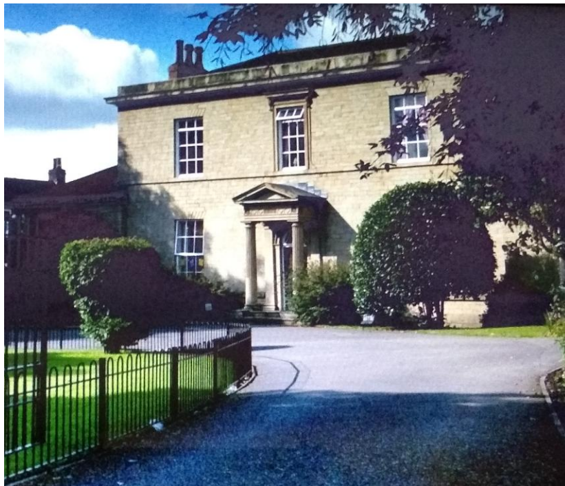
Springstone House July 2000 Copyright IoE Mr John Ulrick. Source Historic England Archive
