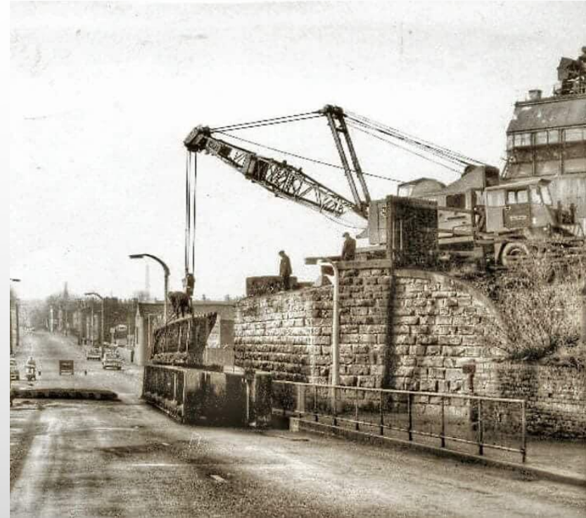
Railway Bridge being demolished
